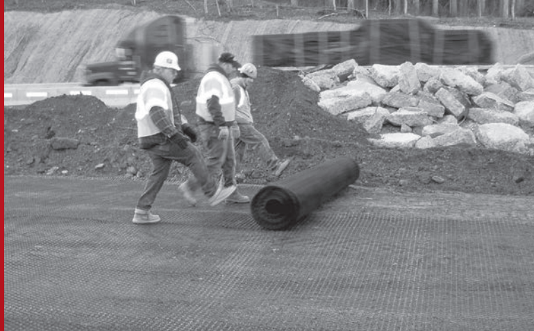
Rolling out Tensar® Geogrid.
