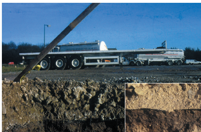
After 11 years of traffic in a truck park, the boundary between the base and subgrade remains distinct. Tensar Geogrid is the only material used to separate the base and the subgrade.
