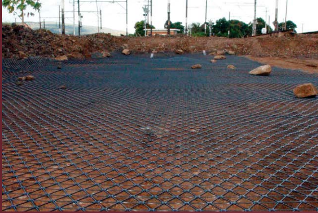
IMAGE C: To stabilize the sub-ballast under a new rail line, geogrids are simply rolled out directly on top of the prepared subgrade.
