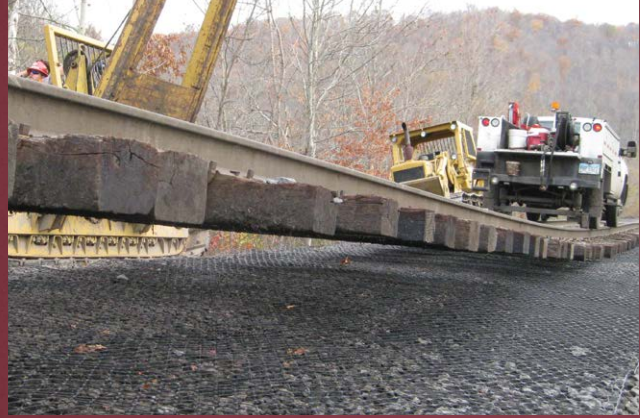
IMAGE D: Existing track can be jacked up so that new geogrid and ballast can be added.
