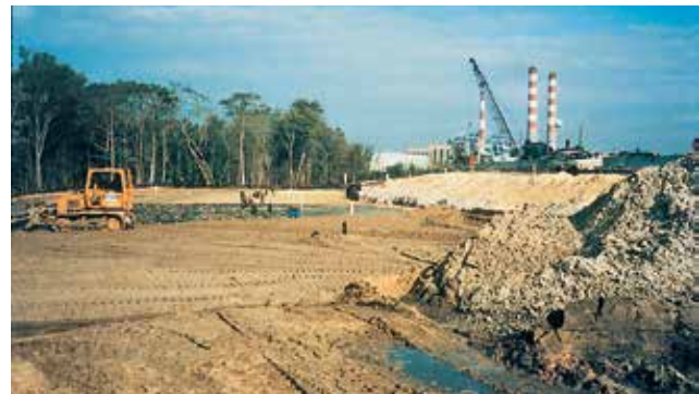
Bridge Approach – State Road 15/US 17, Florida
