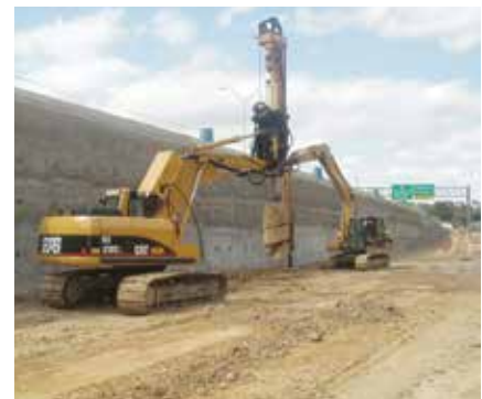
Sam Houston Tollway Widening - Texas
