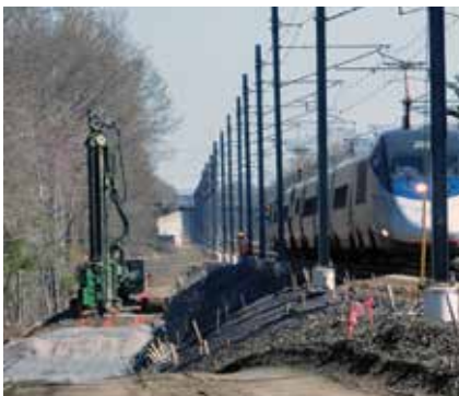
Retaining Wall and Railroad Line – Rhode Island
