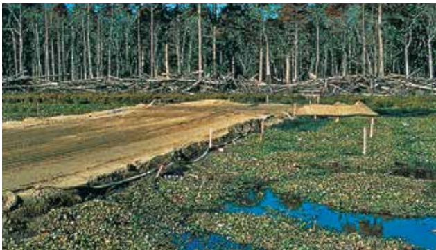
Westminster Levee – Jefferson Parish, Louisiana
