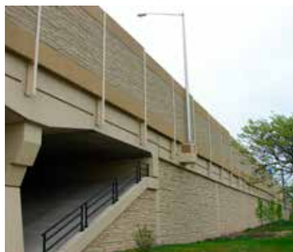
MSE Walls And Embankments - Wisconsin
