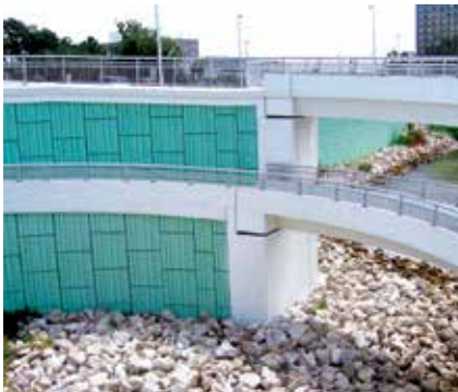
Memorial Causeway - Clearwater, Florida
