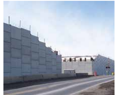
County Road 124 Overpass - Delaware County, Ohio
