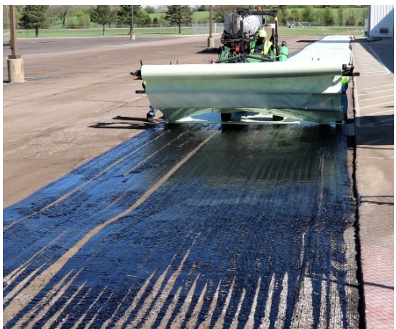
Example of too light of asphalt binder
