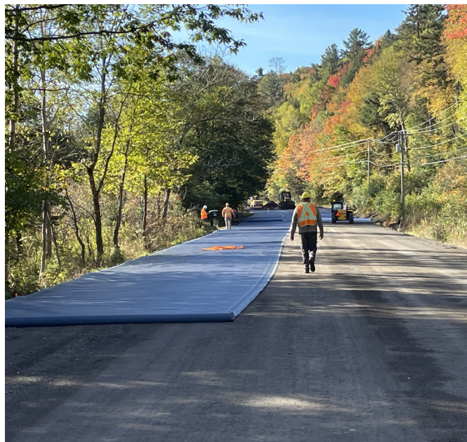
Image 1: MIRAFI H 2 Ri installed parallel to planned traffic flow over a prepared subgrade
