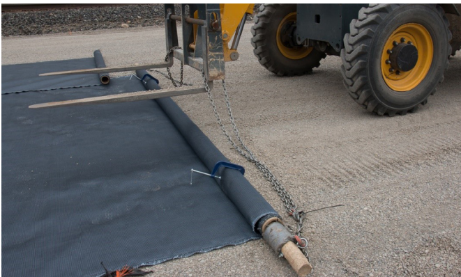
Image 15: Clamps used to secure the material to the core
