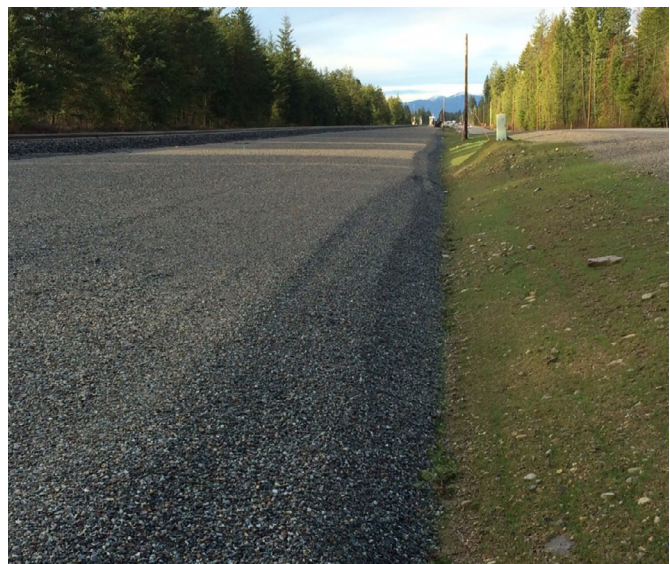
Image 10: Water movement with edge termination
