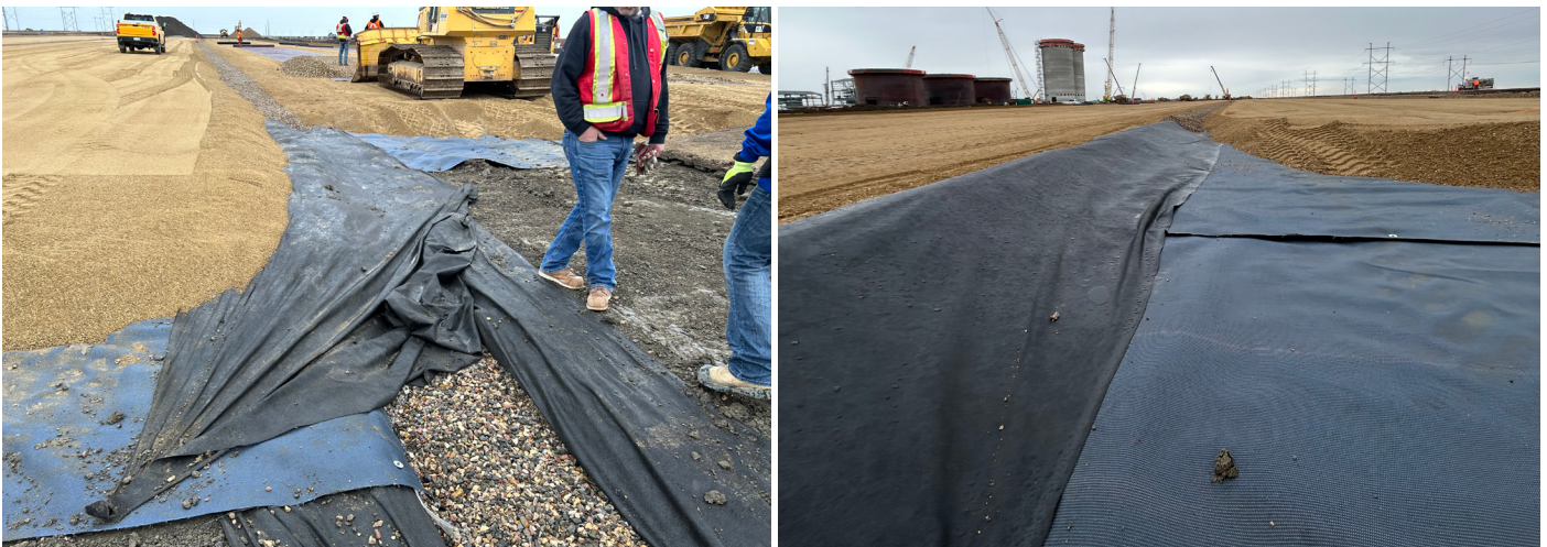
Image 12: MIRAFI H 2 Ri termination into edge drain
