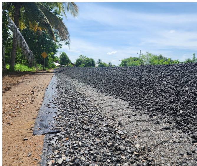
Image 9: Daylighting installation using Rip Rap to cover the exposed edge of MIRAFI H 2 Ri
