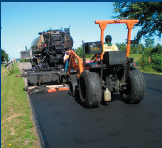
INSTALL FABRIC OVER LIQUID ASPHALT
