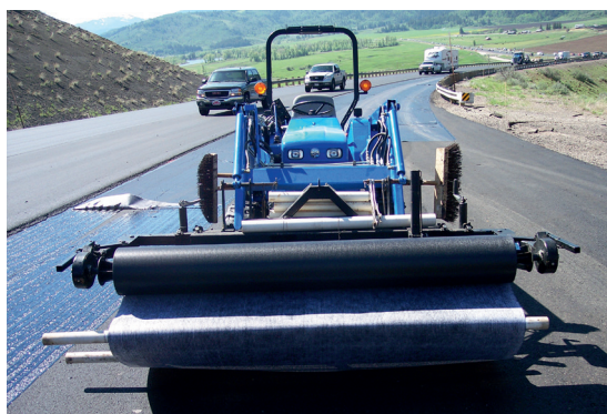
GlasPave is easy to install using conventional equipment.
