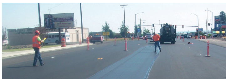
The higher strength at low strain of GlasPave Paving Mats extends pavement life by delaying reflective cracking.
