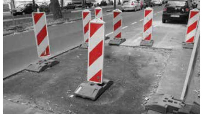
Fast and effective full depth patch repair.
