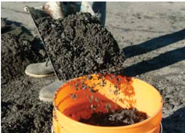
IMAGE A: Milled asphalt containing GlasGrid product can be easily recycled for use on other projects.
