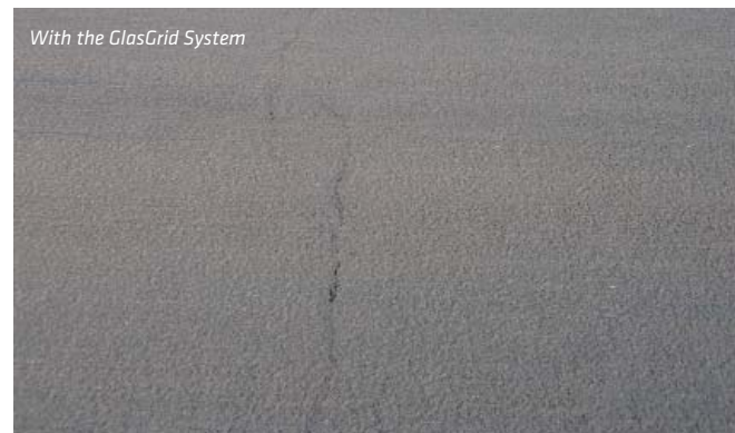
Pavement surface condition following 11 years of post-rehabilitation service.
