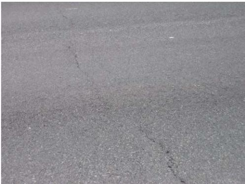
Figure 2: Recommended Application rate - 0.25 gal/yd<sup>2</sup>
