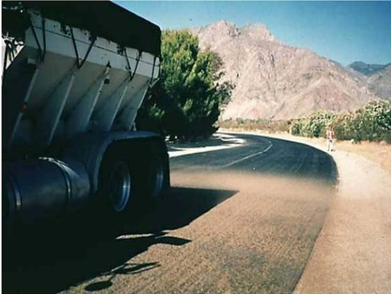
Figure 9: Spreading sand
