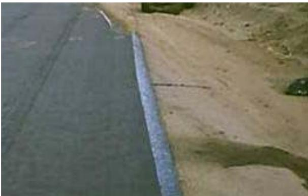
Figure 4: Tack coat spray width beyond fabric
