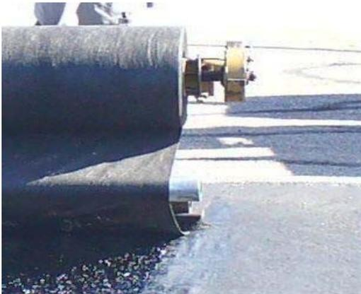
Figure 7: Longitudinal overlap
