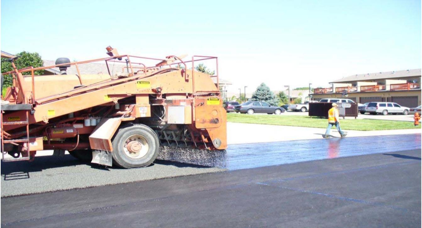
Figure 12: Chip seal installation over installed paving fabric
