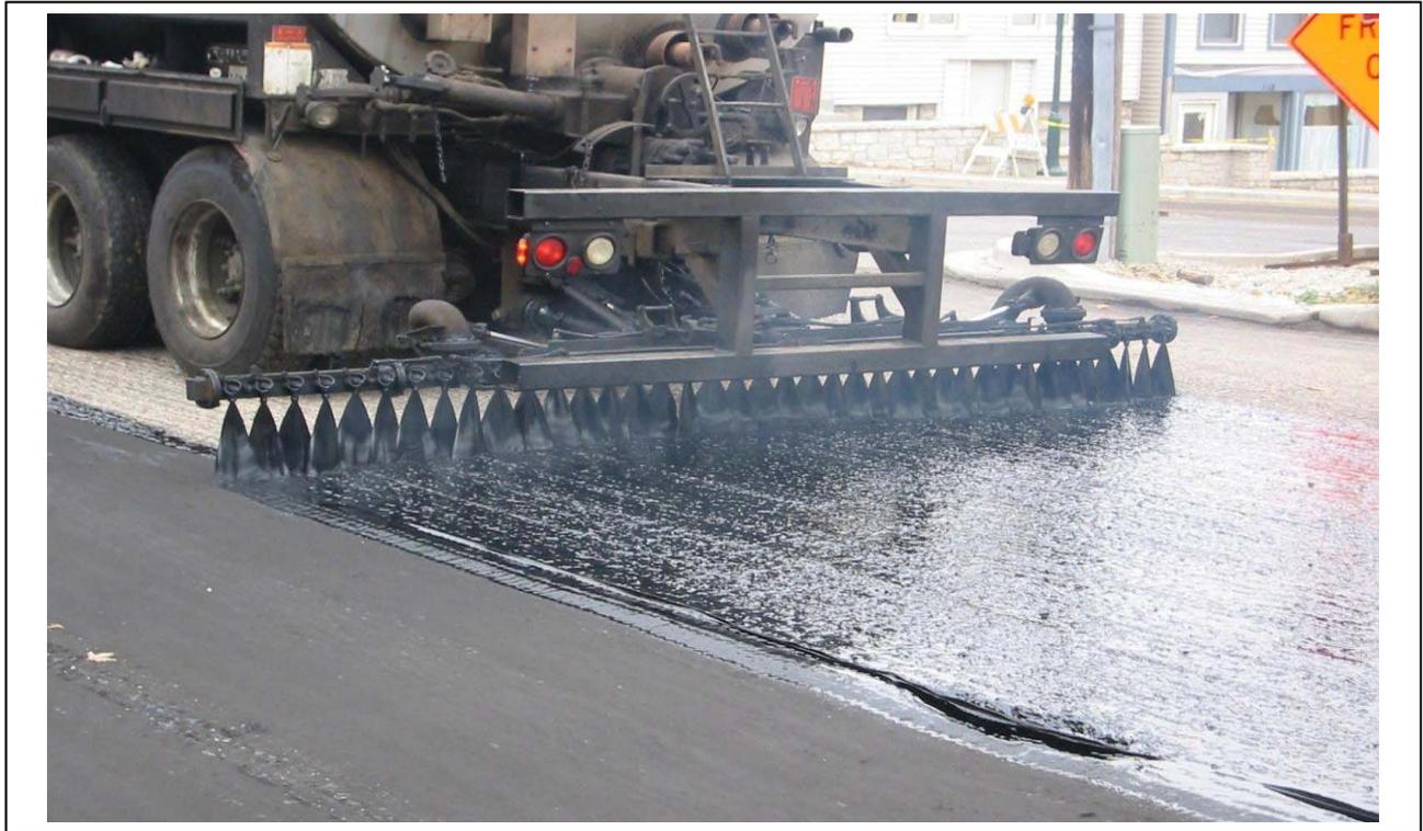
**Figure 1: Tack coat being applied.**
