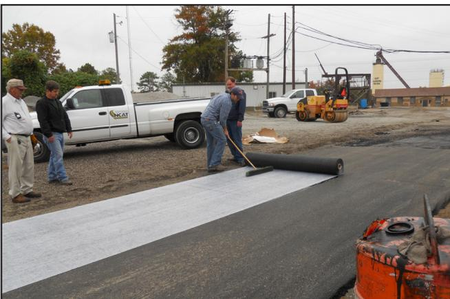
Figure 1 Installation of GlasPave fabric on a test section at East Alabama Paving.
