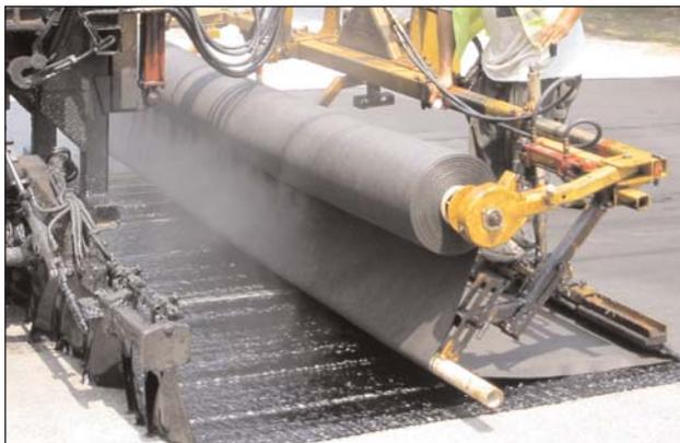
After the asphalt cement was applied to the existing pavement, Mirapave® 500 was installed.
