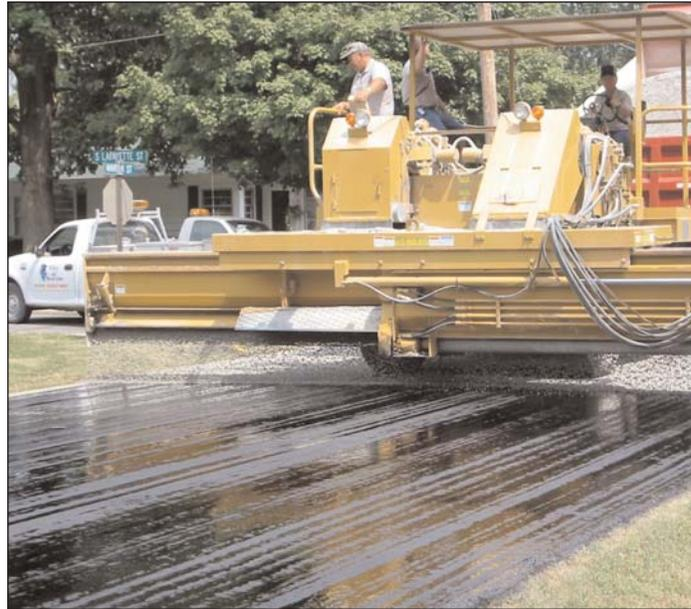
The chip seal aggregate was applied using a variable width spreader.
