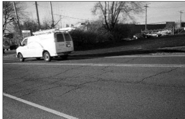
Older roads within the area that lack paving fabrics suffered from unnecessary cracking and deterioration.
