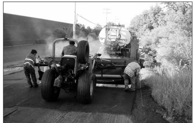
Mirapave® 700 was installed, and a polymer asphalt binder was used in this installation.
