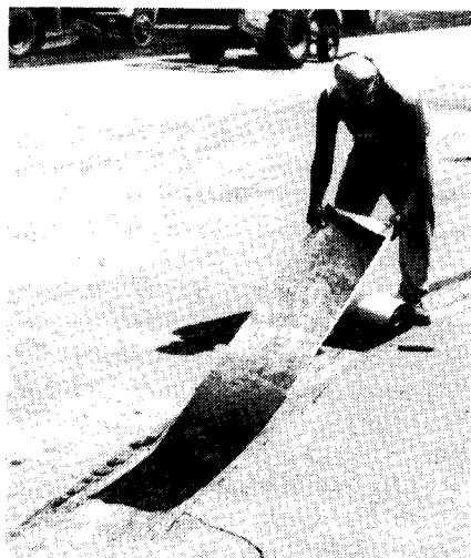
Twelve-inch strips of Petrotac were quickly installed to dissipate the stress that causes reflective cracking and to provide waterproofing benefits.
