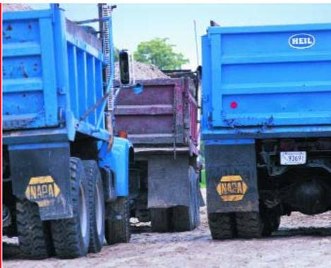
The initial lift of sand received repeated trafficking by fully loaded dump trucks.
