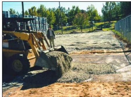
A storage yard for the plant is created by applying a single lift of GAB atop Tensar BX Geogrid laid over “Georgia Red Clay”.
