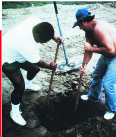
After completion of the sand construction, for both the access road and the mainline levee, excavations were made to install monitoring devices.
