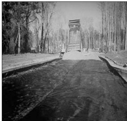
Mirafi ® 500X used for separation under residential street
