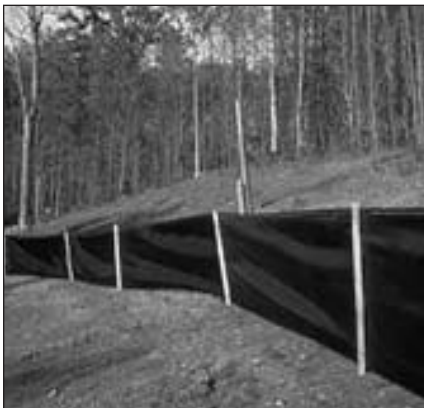
Mirafi ® Silt Fence with posts used for sedimentation control
