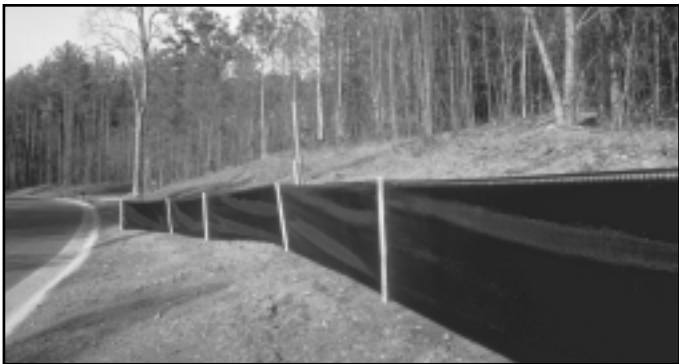
Mirafi® Silt Fence used in erosion control application.
