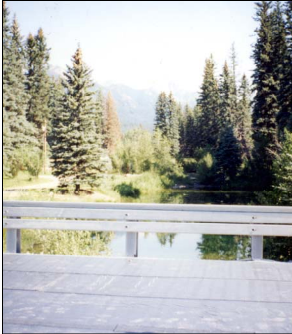
Bridge Decks and Parking Garage Applications
