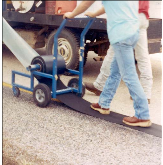
Parking Lots, Pavement Joint & Crack Applications
