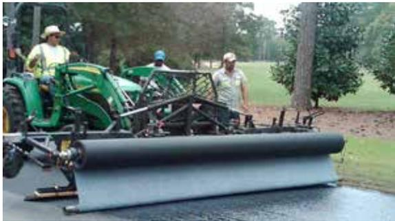
*Image 1: Interlayer laydown equipment.*
