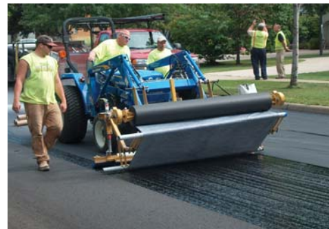
GlasPave50 is easy to install and does not shrink like conventional paving fabrics.
