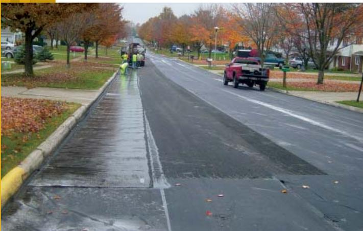
Indeed, tack coats help prevent debonding between courses, slippage of installed interlayers and even surface cracking to strengthen pavements and extend their performance life. But conventional tack coats present their own set of challenges as well:
