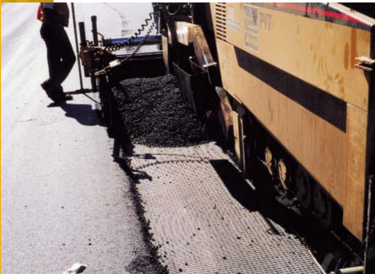
Both products are suitable for construction and rehabilitation.
