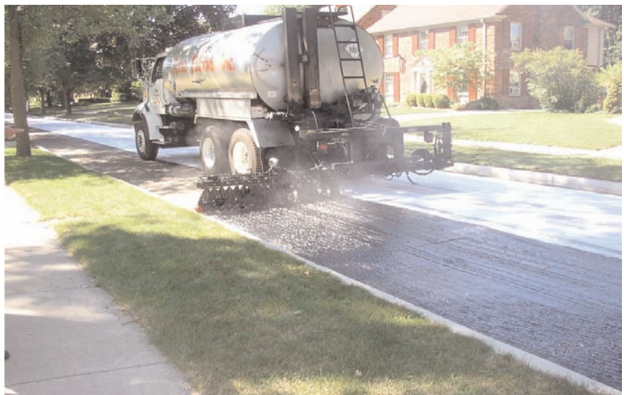
TruPave® installation, showing the application of hot asphalt tack and TruPave® installed on the adjacent lane. Hot asphalt tack also serves as a "crack filler" on small to micro-cracks on the existing surface.
