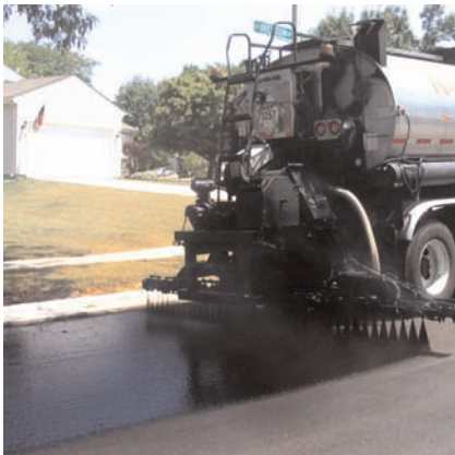
PG70-26 modified with SBS polymer was spread at a rate of .32gal/yd 2 .
