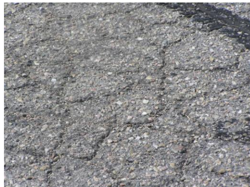
Figure 3: Application rate - .33 gal/sy
