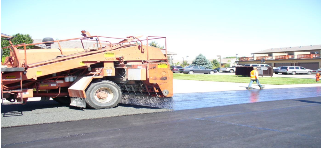
Figure 12: Chip sealing over paving fabric
