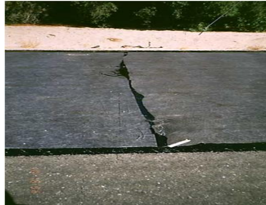
Figure 8: Transverse joint
