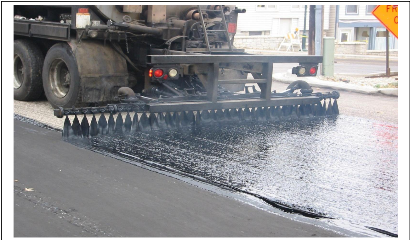
Figure 1: Tack coat being applied
