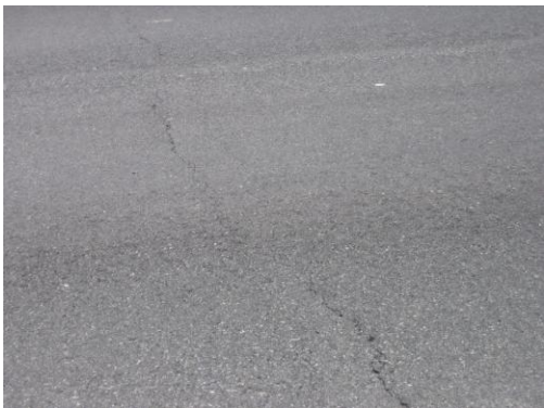
Figure 2: Application rate - 0.25 gal/sy
